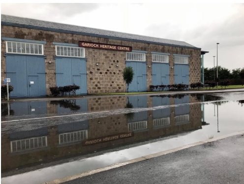
Flooded grounds of Garioch Heritage Centre in July 2020
